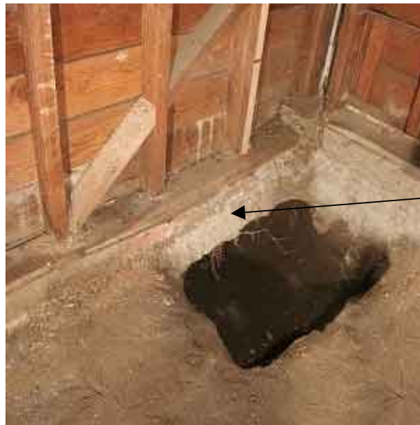
Old Foundation, 6 inches tall, 4 inches embedment, 10 inches wide.
