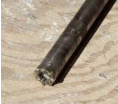
Figure 6. The crew hit rebar while drilling holes for new anchor bolts. Since moving the holes was not an option, they used this special rebar drilling bit from Simpson to cut through the metal.
