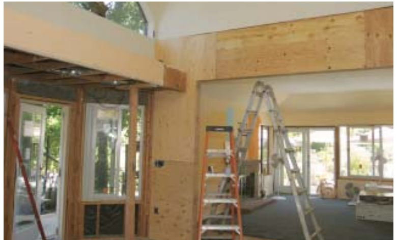
Figure 10. The crew completed the structural work by studding in the panels (left) and replacing the missing plywood shear sheathing on the kitchen side of the wall (above).
