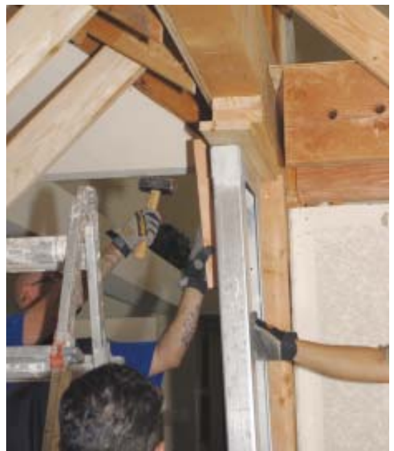
Figure 8. A carpenter places a required steel bearing plate (above) over anchor rods glued in the previous day. The panel will fit over the rods and land on the plate. At right, the crew wedges the top of the panel against solid blocking on the underside of the header.
