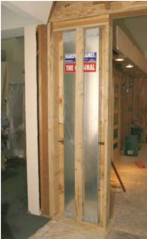
Figure 10. The crew completed the structural work by studding in the panels (left) and replacing the missing plywood shear sheathing on the kitchen side of the wall (above).
