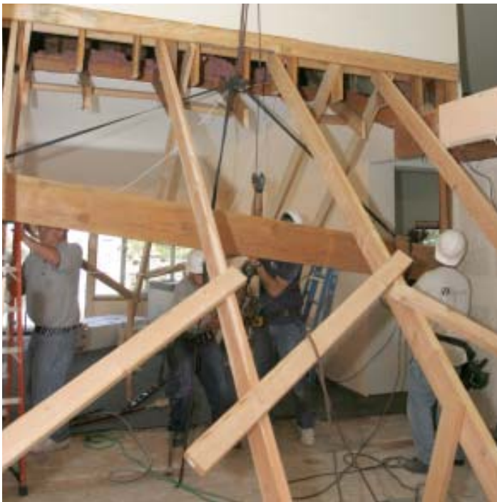
Figure 5. The crew used a block and tackle (above) to hoist the header high enough to get a worker's shoulder under one end and lift it onto a jack stud. With cripples bearing down on the header along its span, it was necessary to wedge the other end of the header into position by beating the angled jack stud in with a sledge (right).
