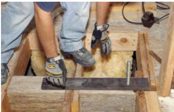
Figure 8. A carpenter places a required steel bearing plate (above) over anchor rods glued in the previous day. The panel will fit over the rods and land on the plate. At right, the crew wedges the top of the panel against solid blocking on the underside of the header.
