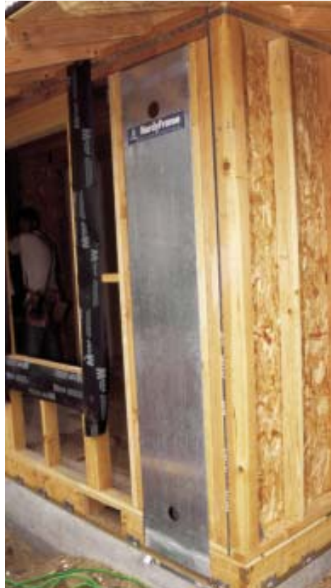
Figure 3. Manufactured shear panels are made from either steel or a combination of wood and steel. At far left, Simpson's Wood Strong-Wall panel strengthens and stiffens a wall containing a garage-door opening — a common application. In the project at left, a Hardy panel allows the contractor to include more window area than would be possible with conventional shear walls. In these installations, the panels sit on a mudsill or directly on the foundation.
