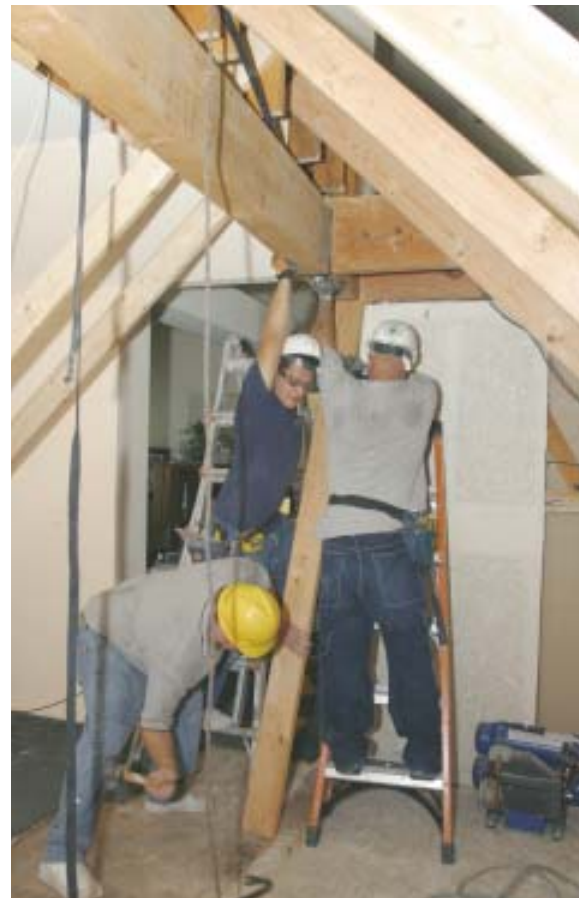
Figure 5. The crew used a block and tackle (above) to hoist the header high enough to get a worker's shoulder under one end and lift it onto a jack stud. With cripples bearing down on the header along its span, it was necessary to wedge the other end of the header into position by beating the angled jack stud in with a sledge (right).
