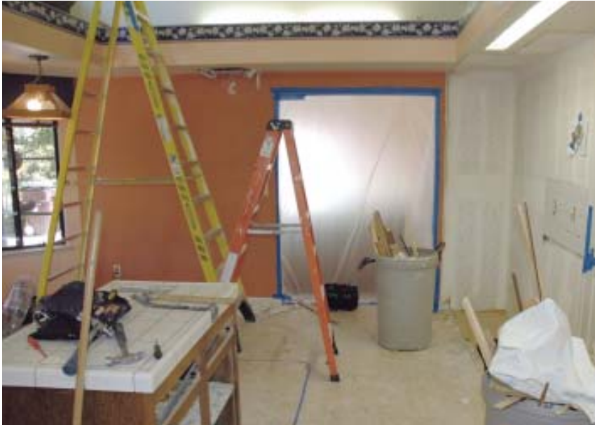
Figure 1. In the original house, built in the 1980s, a 5-foot-wide doorway linked the kitchen and family room; the author suggested enlarging this opening.
