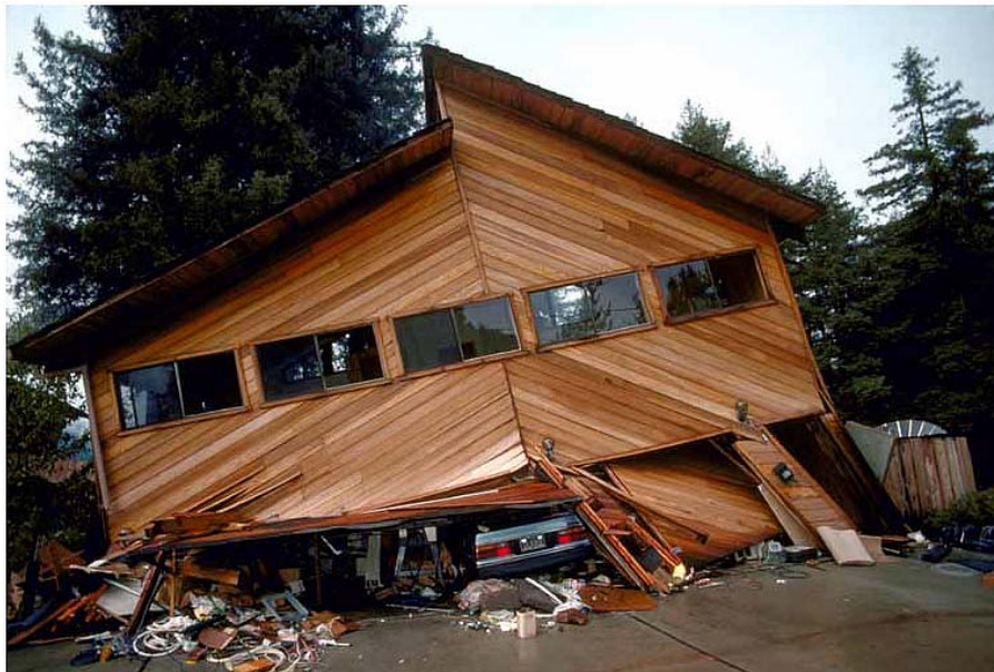
The narrow tall shear walls on this house tipped over.
