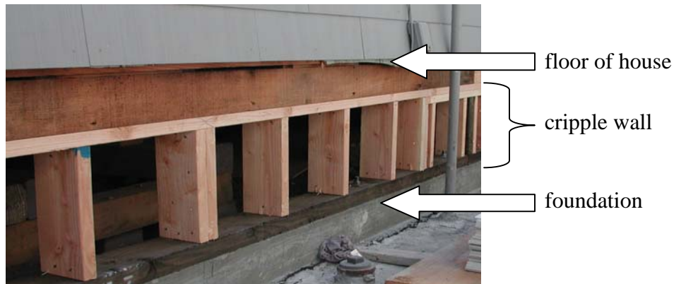
A typical cripple wall seen from the outside Photo courtesy Summerfield Inspections, Berkeley
