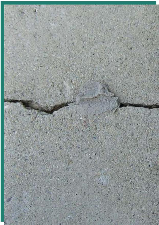
Figure 2: Mortar Thumbprint Crack Monitor
