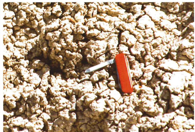
(Left) Large cracks in soil indicate extensive drying and shrinking of expansive clay. This type of crack appears during dry seasons. (Photo by Raymond C. Harris)
