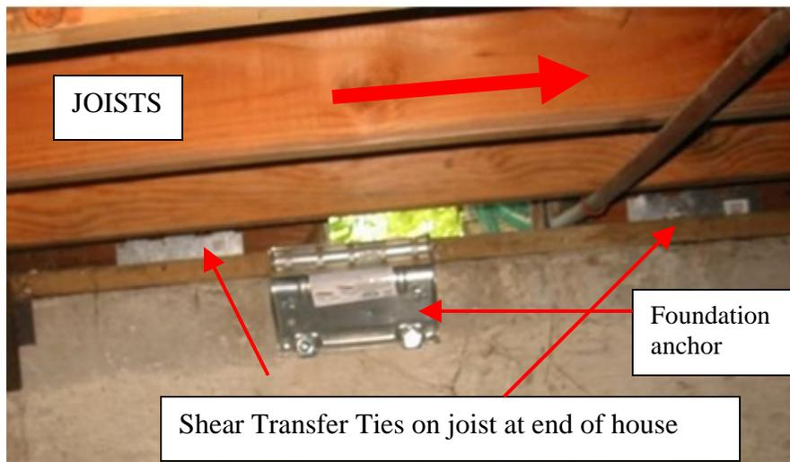
Here is a photo of floor joists that run parallel to the foundation. The joist sitting on the mudsill at the far end that has the foundation anchor attached to it is probably not adequately nailed and can slide off the mudsill and damage the house. This condition normally occurs on the front and back of the home and shear transfer ties are required.
