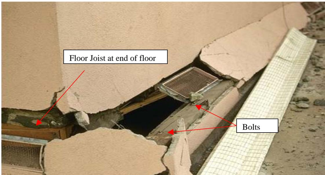
Here is an example of a failure when the floor slid off of the bolted mudsill. This is prevented with shear transfer ties. This failure occurred on the short side of the house.
