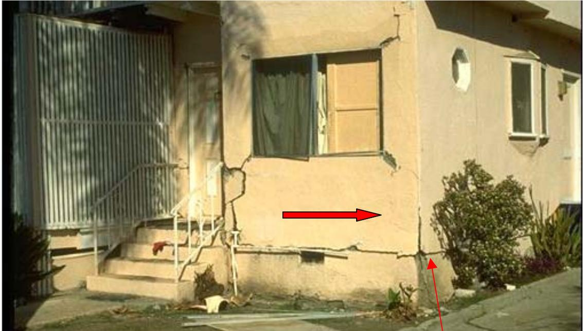
Here is an example of another bolted house where the floor framing (floor joists) sitting on top of the foundation moved but did not slide off. The entire house shifted to the left and caused the front window break. The failure occurred on the short sides of the house.
