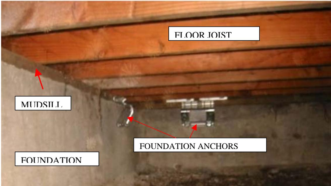
Foundation Anchors are bolted to the side of the foundation and mudsill. The mudsill is one part of the floor that can slide in an earthquake.
