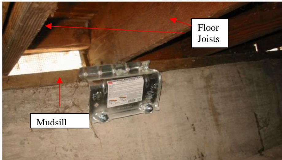
When the floor joists are perpendicular to the mudsill (usually the long sides of the house) they are almost always adequately nailed to the mudsill and no shear transfer ties are needed. This is because adequate nailing must be done as part of the construction process.
